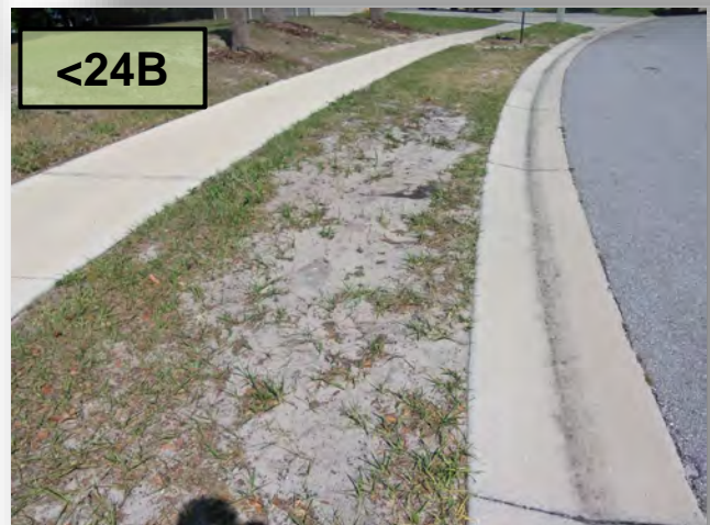
24. Hanover Drive: Damaged turf and exposed sand were observed in the east and west side easements across from the retention area; visible rutting suggests the decline is likely associated with vehicle activity. (Pics 24A> & 24B>)
